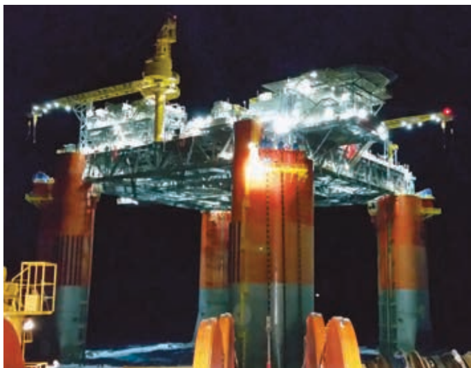
Figure 7. Delta House FPS as seen at night from back deck of an AHV.
