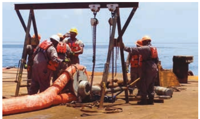
Figure 5. Connecting large polyester rope segment to mooring chain segments.
