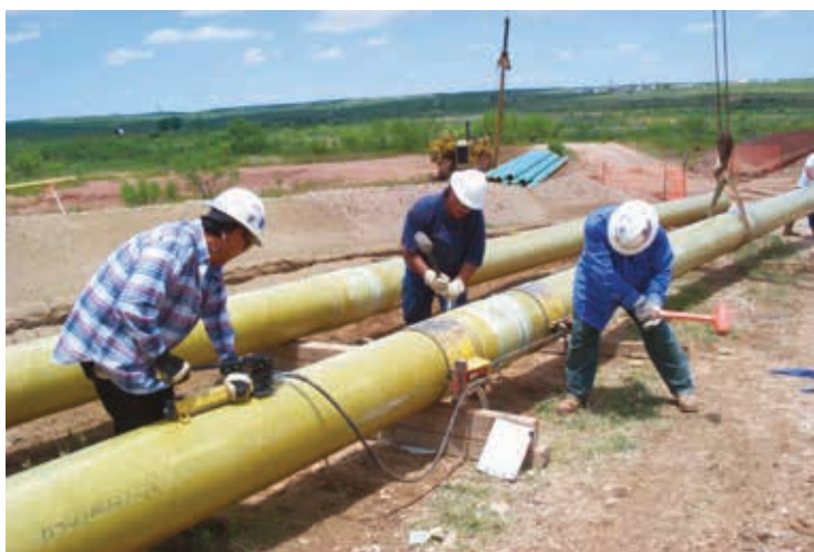
Figure 2. Large diameter Red Thread HP installation.
